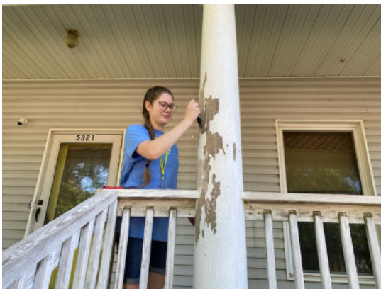
Chipping paint off a porch at 3MT
